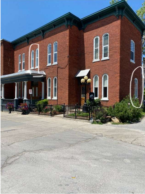
Photo 1. Front Elevation – The windows circled in the photo will be replaced.
