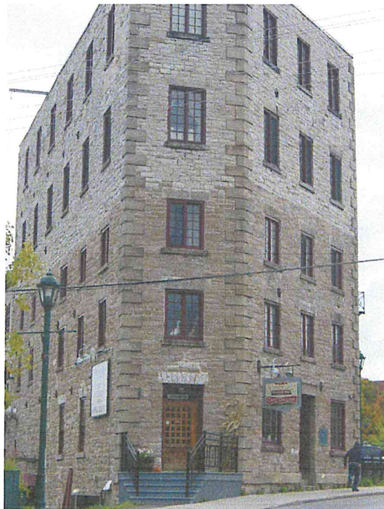
View of Victoria Woolen Mills Building (From Mississippi Mills Web Site)
