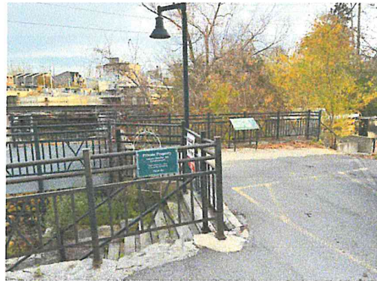
View of Proposed Fence Location Showing Existing Fencing In Adjacent Area
